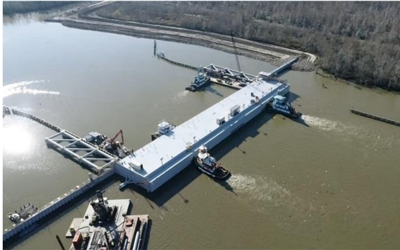
Barge Gate, 446-foot Span
